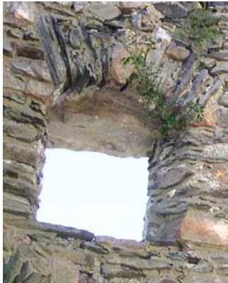
Fig. 5. Window, interior. Photo by Ron Barstad.
